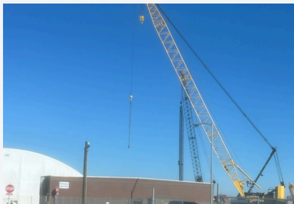
From our jobs: a unit going up under a lattice-boom crane.
